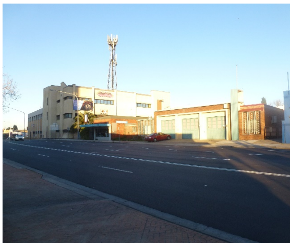
Figure 17: Telstra Exchange building and adjoining retail tenancies to the south
