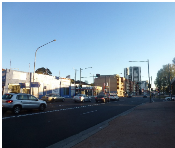
Figure 18: Retail and medium density residential uses fronting Terminus Street to the south
