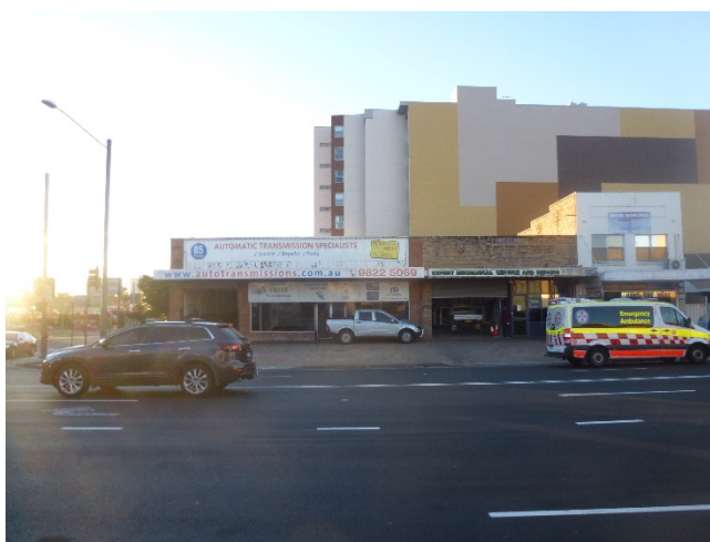
Figure 21: Rear party wall presented to the site
