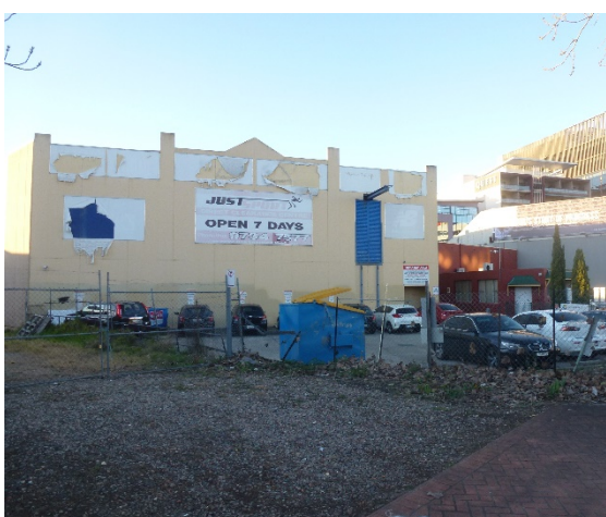
Figure 8: Rear car park of the commercial building as viewed from Terminus Street (south east)
