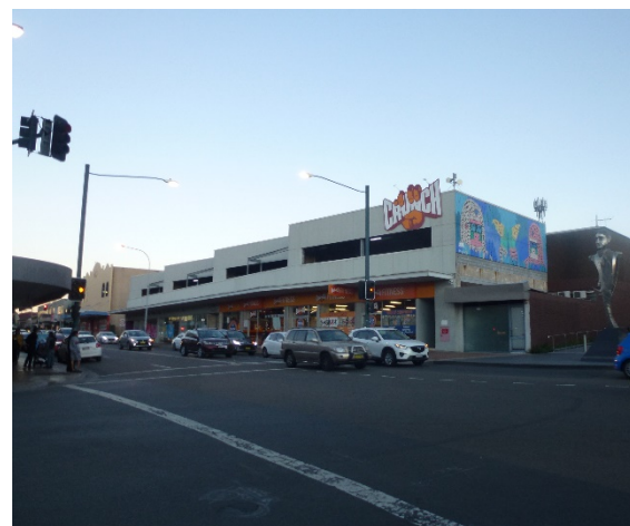
Figure 5: Commercial building occupying the site as viewed from Scott Street (north west)
