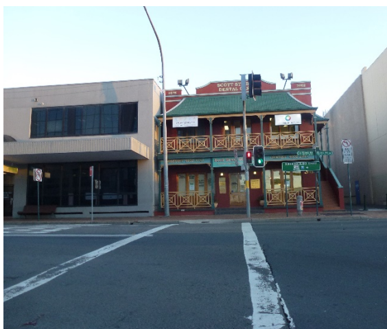
Figure 15: Two storey commercial building to the east of the George Street through site link
